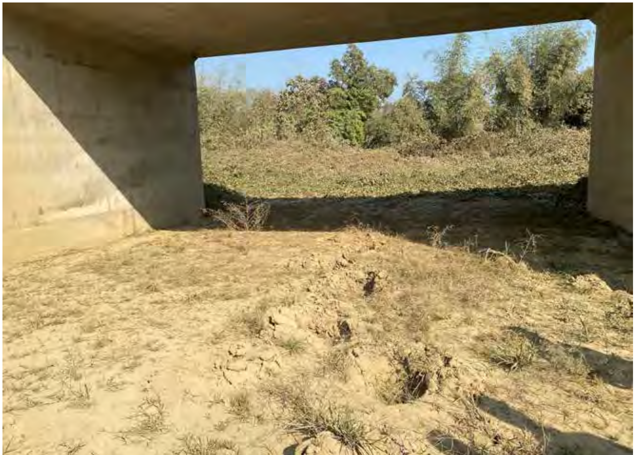
Cox's Bazar railway underpass, Bangladesh. The project increases connectivity between three protected areas that support endangered Asian elephants ( Elephas maximus ). Prints in the ground indicate that elephants are already using the box culvert underpass. © Norris Dodd
