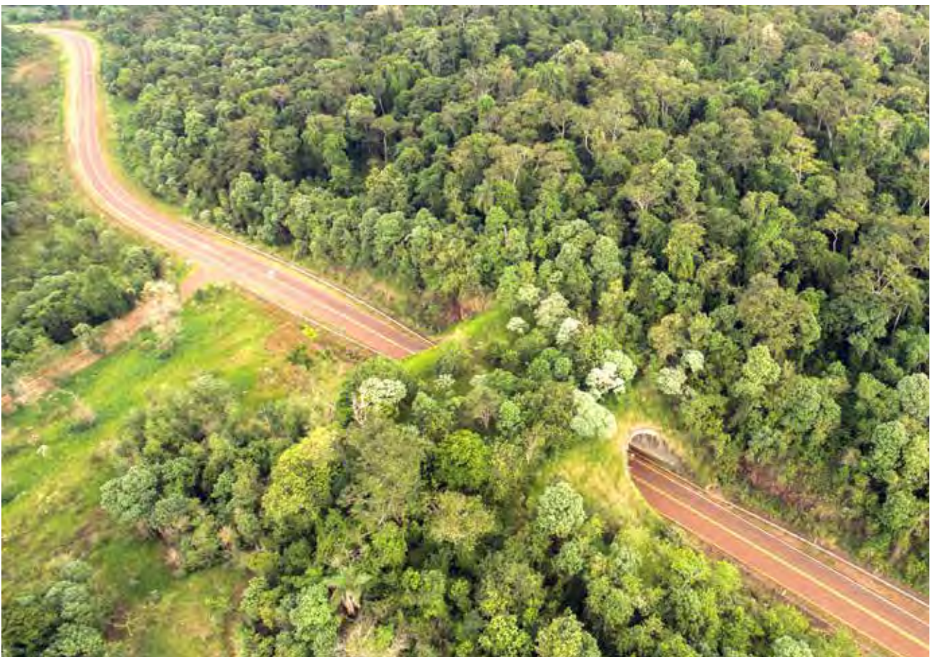
Wildlife overpass across National Route 101, part of the Urugua-í-Foerster Biological Corridor in Argentina © Adobe Stock
