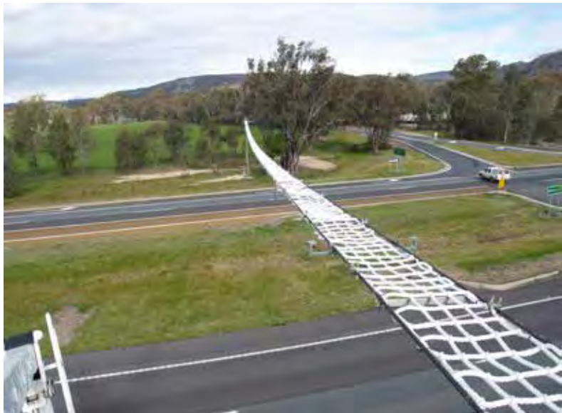
Arboreal crossing over Hume Freeway, Australia © Rodney van der Ree
