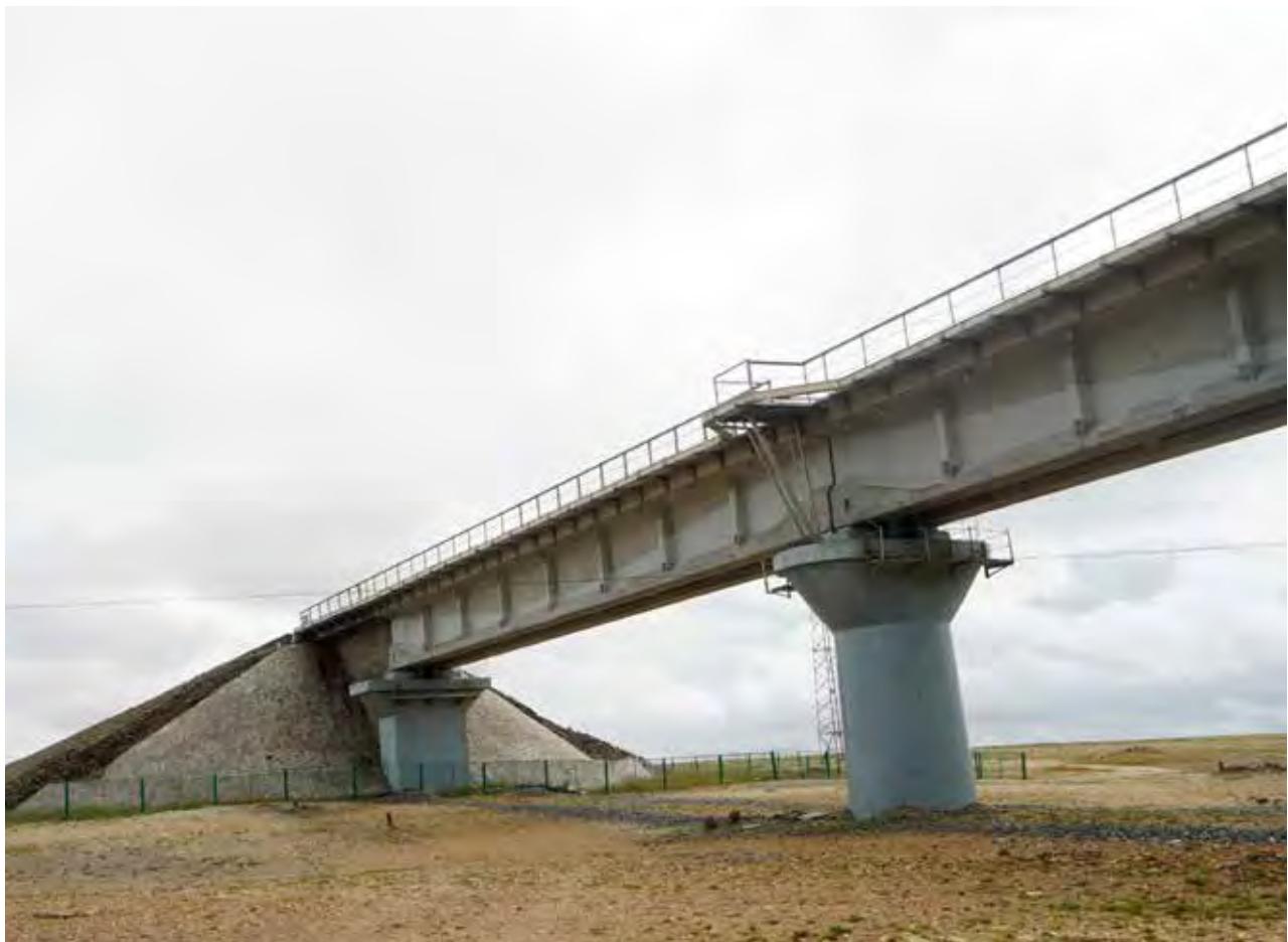
The Qinghai-Tibet Railway (QTR) travels over China's Wubei Underpass, constructed to facilitate Tibetan antelope ( Pantholops hodgsonii ) migration between key habitats on either side of the rail. © Wenjing Xu
