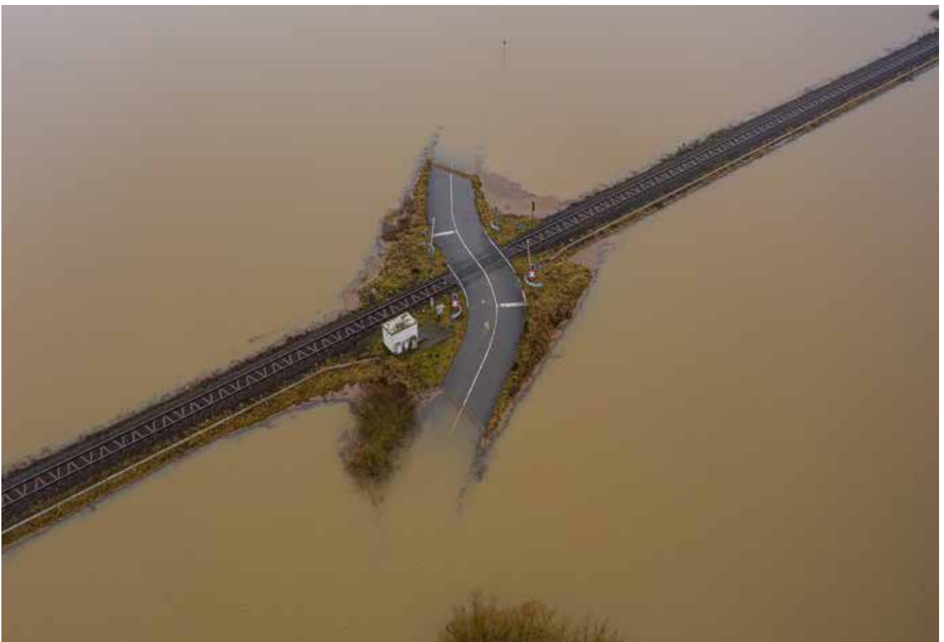
Flooded road and rail intersection. Building resilient infrastructure can reduce vulnerability to ongoing and predicted catastrophic threats of climate change. © Adobe Stock
