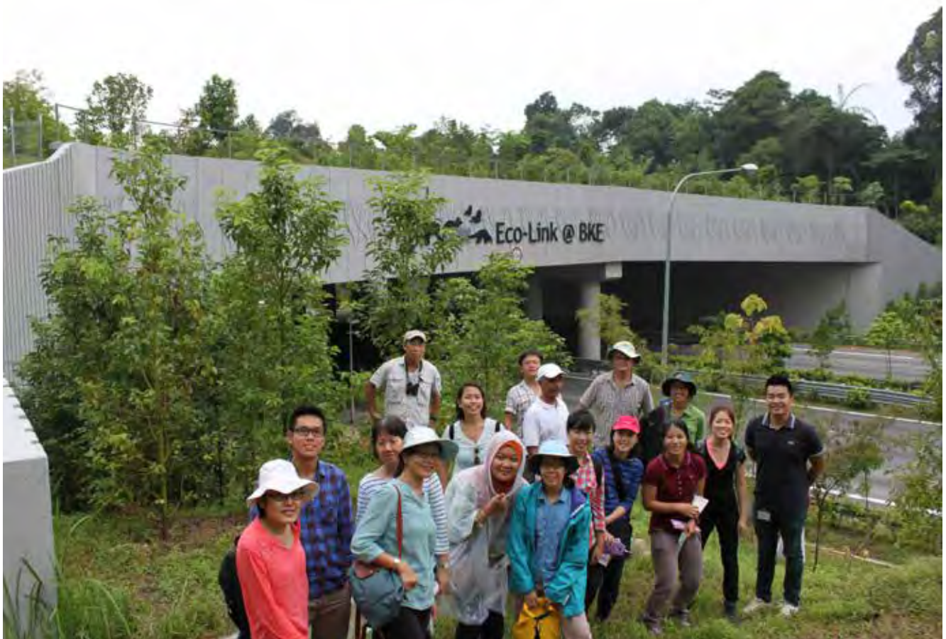
Community members gather to celebrate one of the first wildlife overpasses in Asia, the 140m-long and 44m-wide Mandai Eco-Link@BKE ecological bridge in Singapore. Covered with native plant and tree species and incorporating specialised fencing, the overpass was designed for use by species such as Sunda pangolins ( Manis javanica ) and Palm civets ( Paradoxurus hermaphroditus ). © Rodney van der Ree
