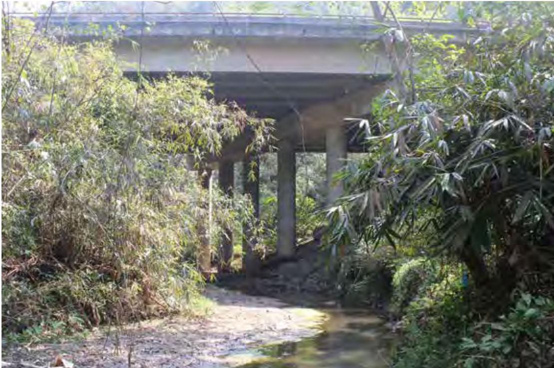
Asian elephant ( Elephas maximus ) underpass across the Sixiao Expressway, Xishuangbanna, China © Yun Wang
