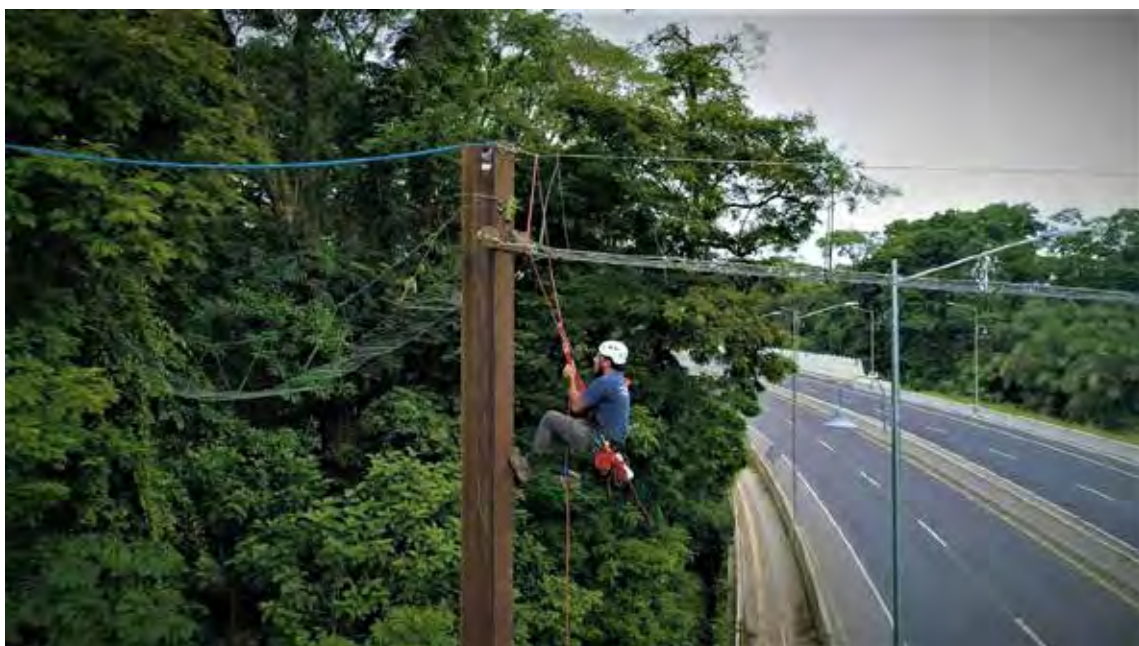
Arboreal species crossing structures are being deployed around the world. Here, a technician in Costa Rica places cameras to monitor their effectiveness and use. © Panthera
