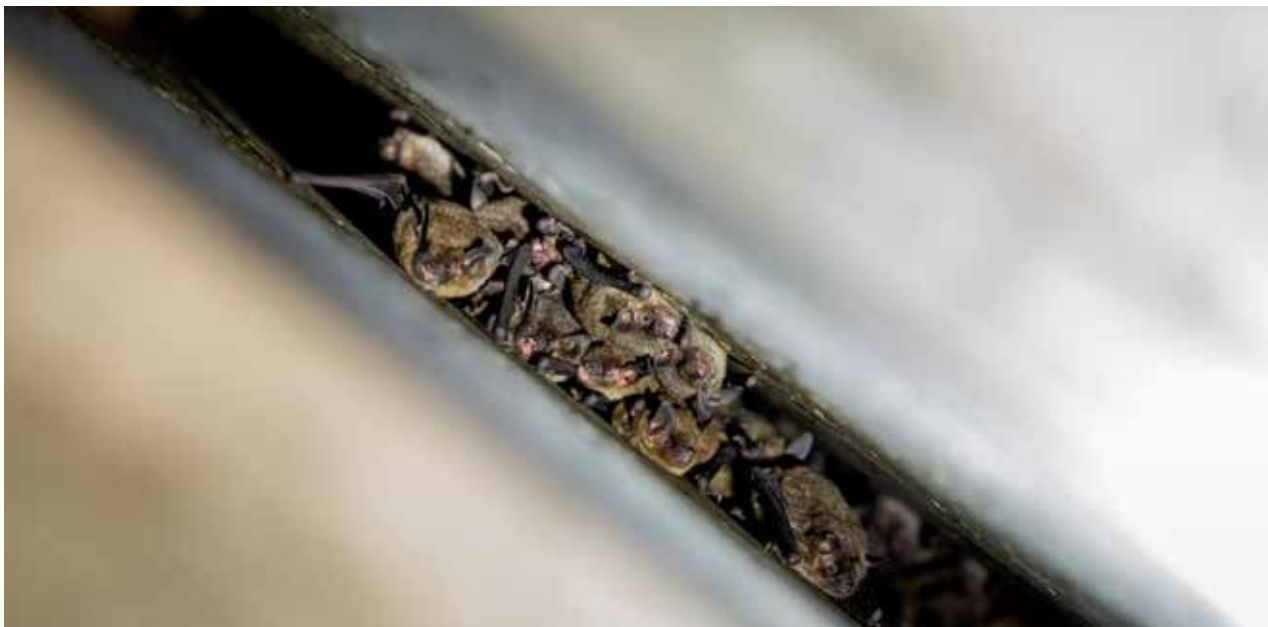
Gray bats ( Myotis grisescens ) roosting between beams on the underside of a bridge in Kentucky, USA. The deteriorating bridge was slated for rehabilitation, but when the bats were discovered, transportation planners adjusted their designs to protect the vulnerable species. Repairs were conducted in midwinter when the bats were hibernating elsewhere. New beams were installed with extra space in between to provide safe habitat for the bats to return. © Kentucky Transportation Cabinet
