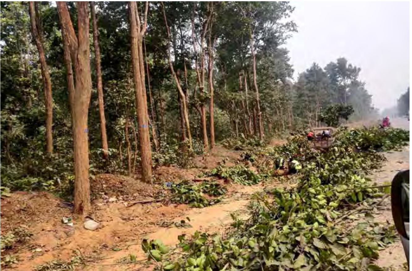
Machinery clearing a forest to make way for the Narayanghat-Butwal Road Project; a 113 km long upgrade of an existing two-lane road to a four-lane highway in Nepal. © Anthony P. Clevenger
