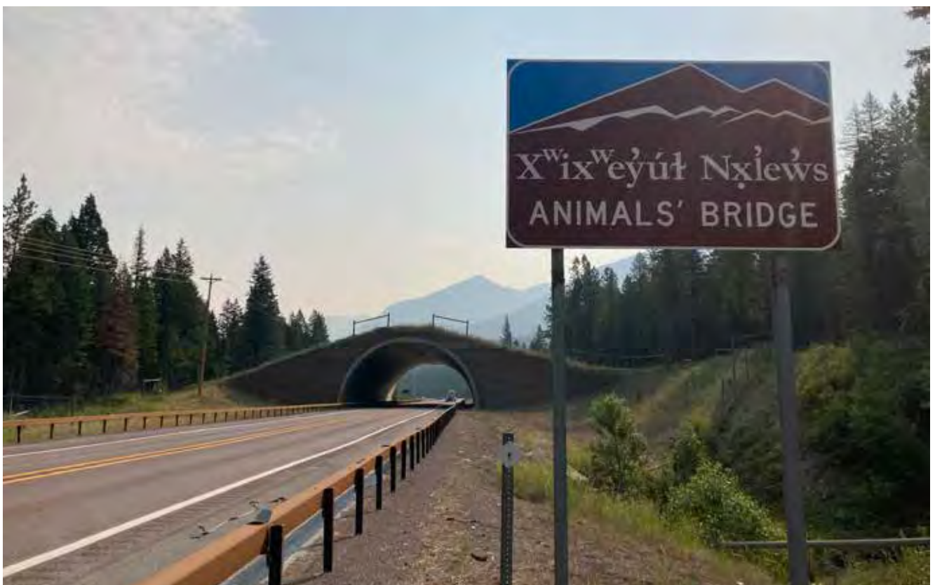
A wildlife overpass and bilingual signage constructed along US Highway 93, which passes through lands of the Confederated Salish and Kootenai Tribes (CSKT) of the Flathead Reservation in Montana, USA. This mitigation measure is one of 41 wildlife crossing structures built along 90 km of road, which makes this area one of the most thoroughly mitigated road stretches in the United States. The Tribes' leadership on the project – and commitment to safety improvements for both motorists and wildlife – grew out of a philosophy that every species has value as an integral part of the whole ecosystem. While collaborating with state and federal agencies, the sovereign CSKT ensured that the project outcomes aligned with their values. © Luca Guadagno
