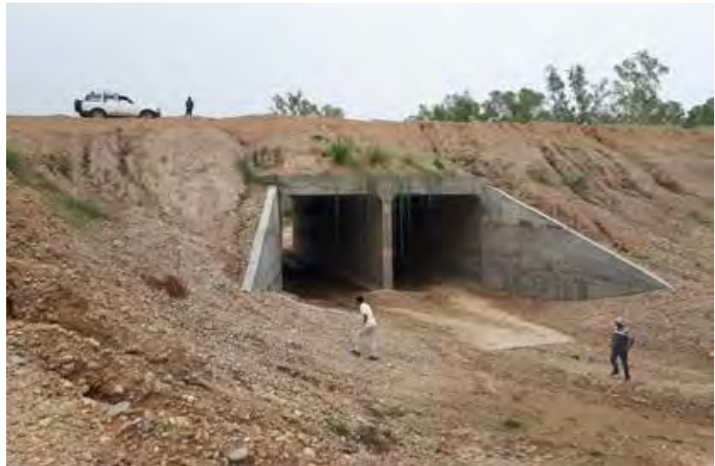
One of 112 wildlife underpasses installed along the 115 km road as part of a revised mitigation strategy for the Narayanghat – Butwal (NB) Road, Nepal © Pramod Neupane
