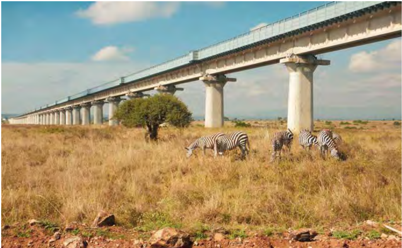
A herd of plains zebra ( Equus quagga ) graze below the Nairobi-Mombasa Railway. Bisecting Nairobi National Park, the rail design allows for wildlife movement under the tracks, but avoidance of the protected area was not taken into consideration. Consequently, the impacts of construction, maintenance and rail effects such as noise, vibrations and movement, are now pervasive. © Martin / Adobe Stock
