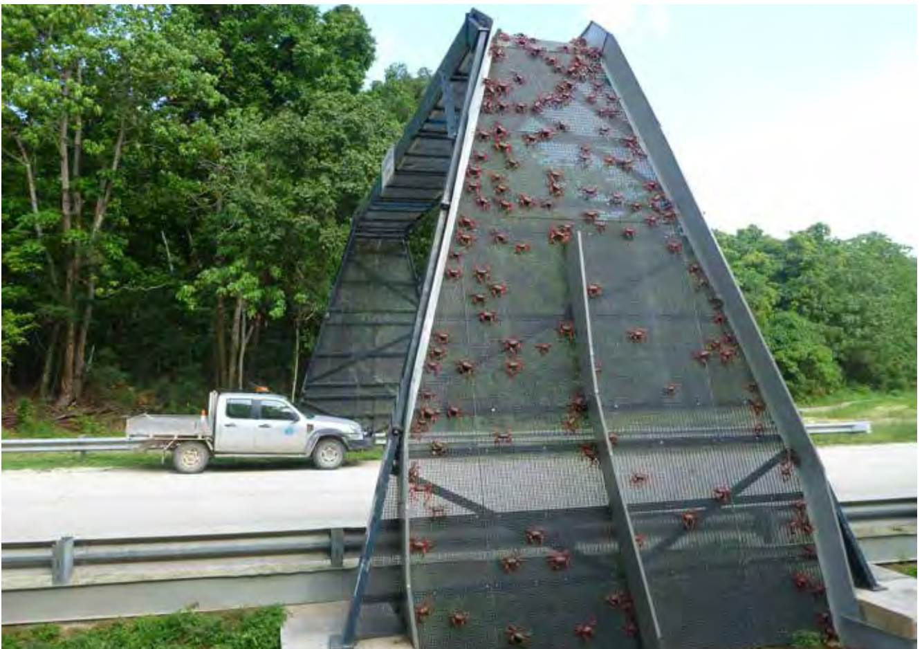
Red crabs ( Gecarcoidea natalis ) use a specially designed bridge with purpose-built directional fencing to safely cross a road during seasonal migration on Christmas Island, Australia. © Parks Australia
