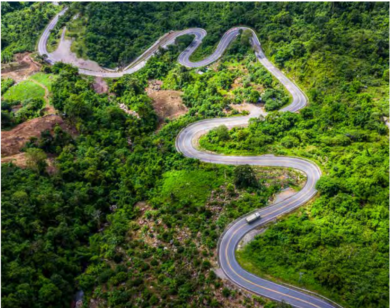
In developing countries, private investors are known to cut construction costs for profit, building deficient infrastructure that over time can require much more maintenance that countries may have to assume. © Adobe Stock
